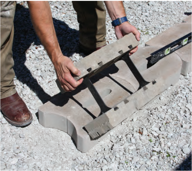
STEP 4: Place the assembled Tandem Wall unit on the top of the U Start Base Block, making sure that the first course is centered on the base block. Check to make sure units are kept level.
