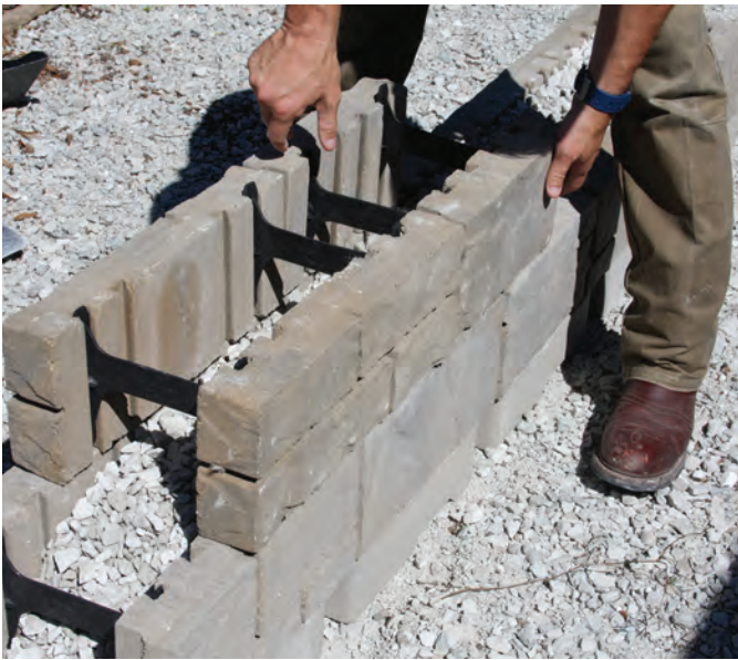
STEP 9: Set additional courses of the Tandem Wall. Making sure that you are keeping the wall in proper alignment. Backfill and compact each additional course.
