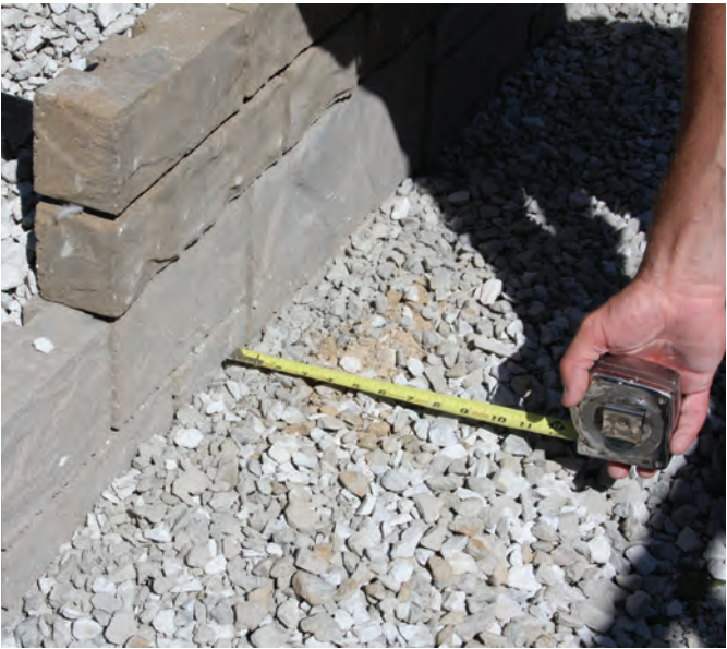
STEP 8: Place 12" of 3/4" drainage rock behind the rear panel of the wall. This will provide for proper drainage behind retaining walls.
