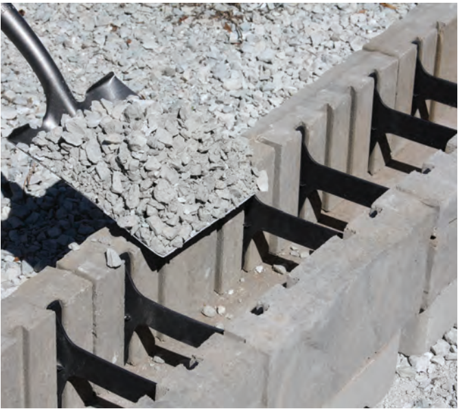
STEP 6: Place 3/4" crushed rock in between the panels to provide frictional connection and proper internal drainage.
