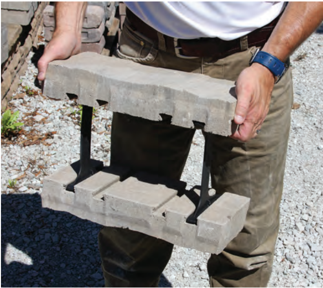
STEP 3: Assemble the Tandem Wall units by inserting the Tandem Wall connectors into the dove tails. Make sure the front and rear panels are the same length.
