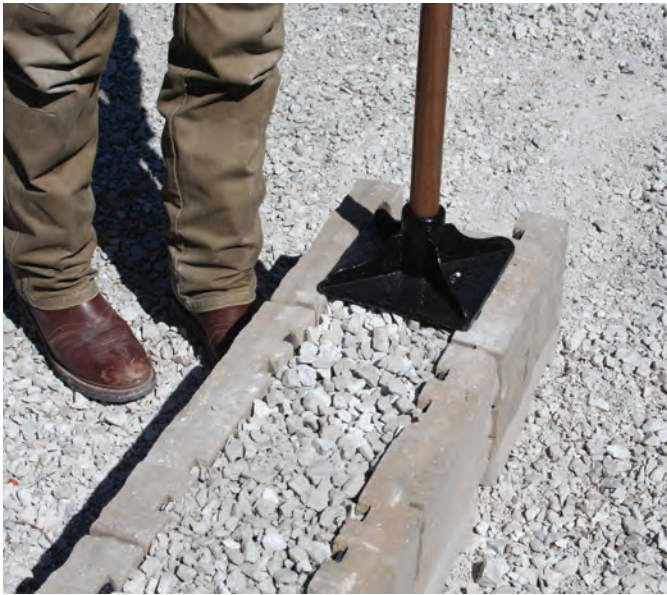
STEP 7: Lightly hand compact the gravel in between the panels for proper compaction.
