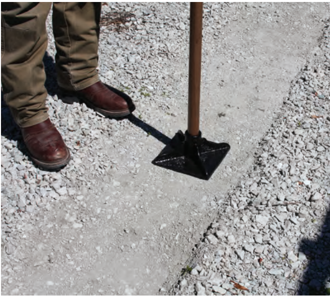
STEP 1: Remove all surface vegetation and debris. Select the length of the wall and excavate a trench the length of the wall and approximately 12" from top of final grade. Then place a minimum of 6" of dense graded aggregate and compact to 95% standard density or modified. It's not recommended to use a pea rock or a rounded type of material on the base.
