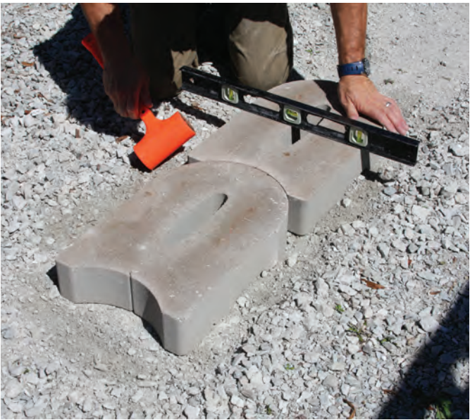
STEP 2: Place the U Start Base Block® on the compacted gravel. Level the U Start units front to back as well as side to side. Making sure the units are fully level.
