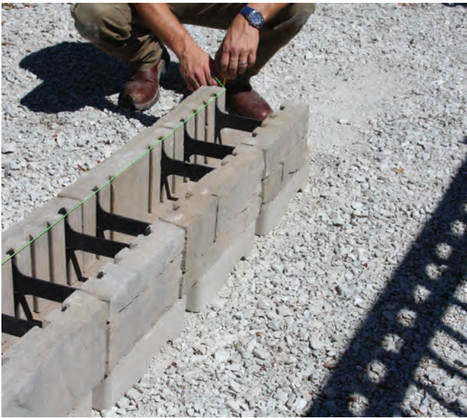
STEP 5: Once the Tandem Wall units have been placed. Run a string line along the back of the front or rear panel to assure you are keeping the wall units straight in line.
