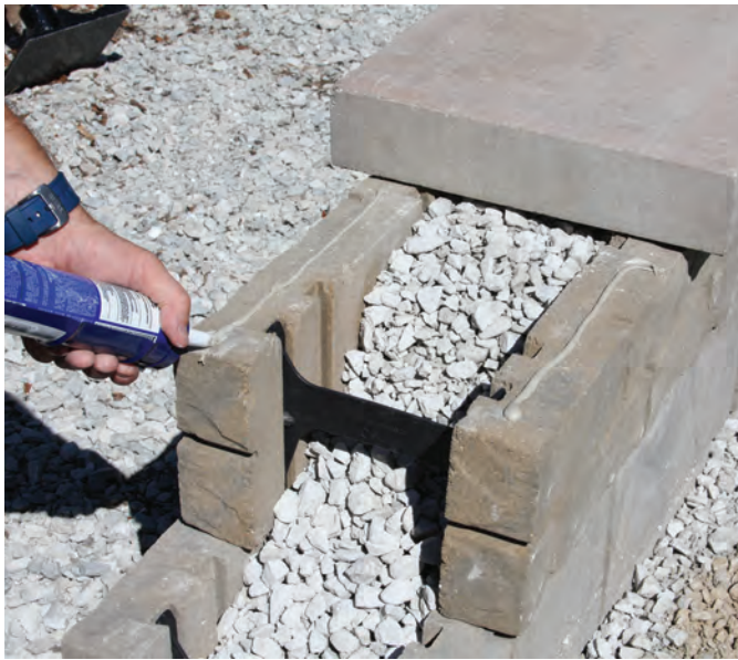
STEP 10: When placing the cap on top of Tandem Wall, use a construction adhesive to secure the cap to the top of the wall.
