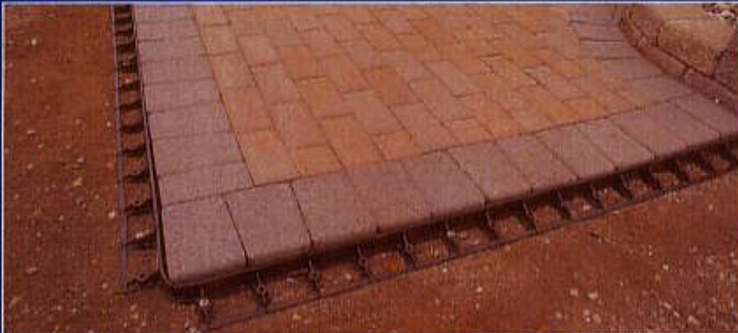
All paver applications require a restrained edge to prevent lateral movement.
